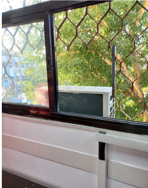
Sawn bars and the danger of falling they pose in a community center in Bat Yam
