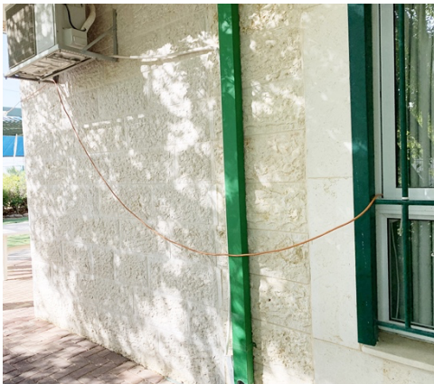
An improvised electrical cable for outdoor lighting at a club for the elderly in Modi'in
